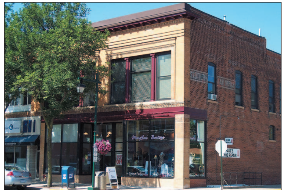
Barry Gillespie of ERA Gillespie Real Estate replaced windows in the apartments above his commercial property at 122-124 N Cedar. Lead paint testing and safety practices were used in the revitalization.
